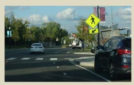
**Pedestrian Refuge Islands (median islands)** – This feature, which is particularly beneficial on wide multi-lane roadways, allows pedestrians to cross a two-way street in two stages by finding a gap in one direction, and then stopping on a median island of sufficient width to wait while searching for a gap in the other direction of traffic.
